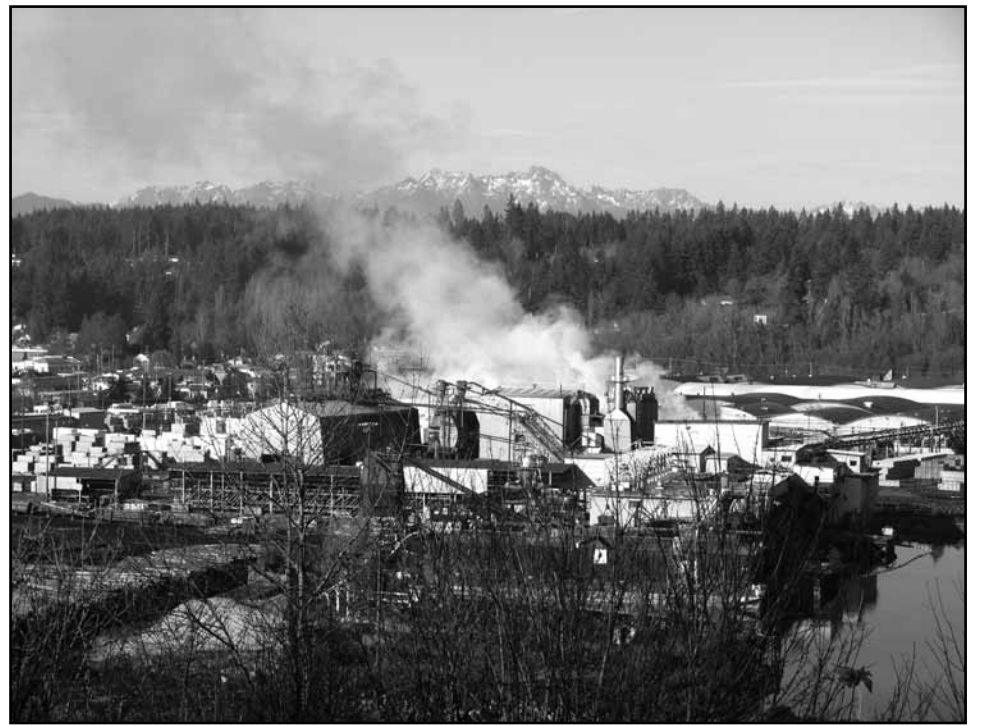
The Simpson lumber mill in Shelton, Wash.
